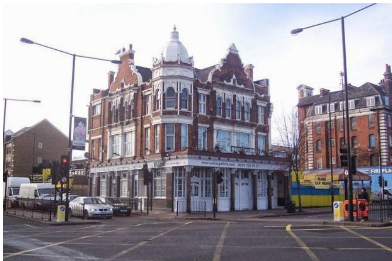
The spot on the Old Kent Road where Penry was executed
